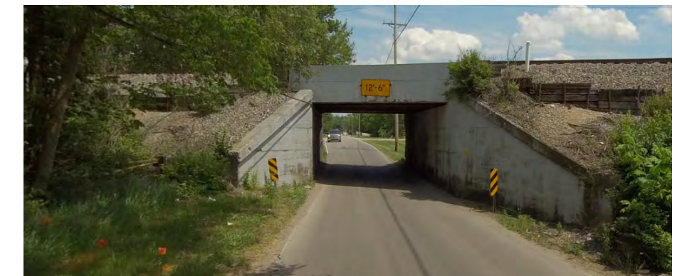
Railroad overpass along Franklin-Trenton Road
